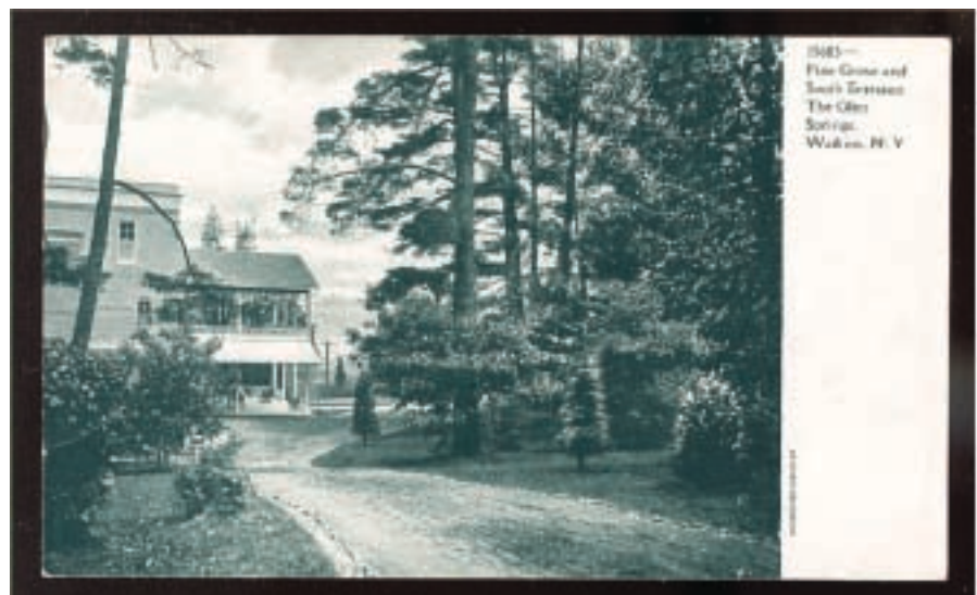
South entrance of the Glenn Springs Hotel
