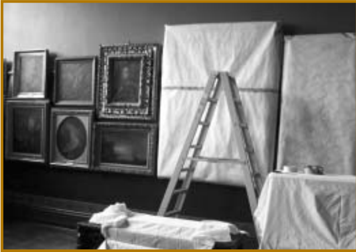
Olana's Dining Room being prepared for systems installation.
