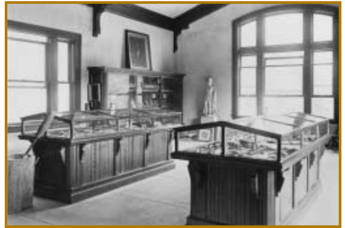
The original installation at William Pryor Letchworth Museum, 1913.
