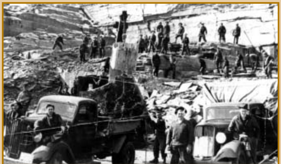
CCC workers excavating stone at a quarry in Montour Falls for Watkins Glen State Park, courtesy Schuyler County Historical Society.
